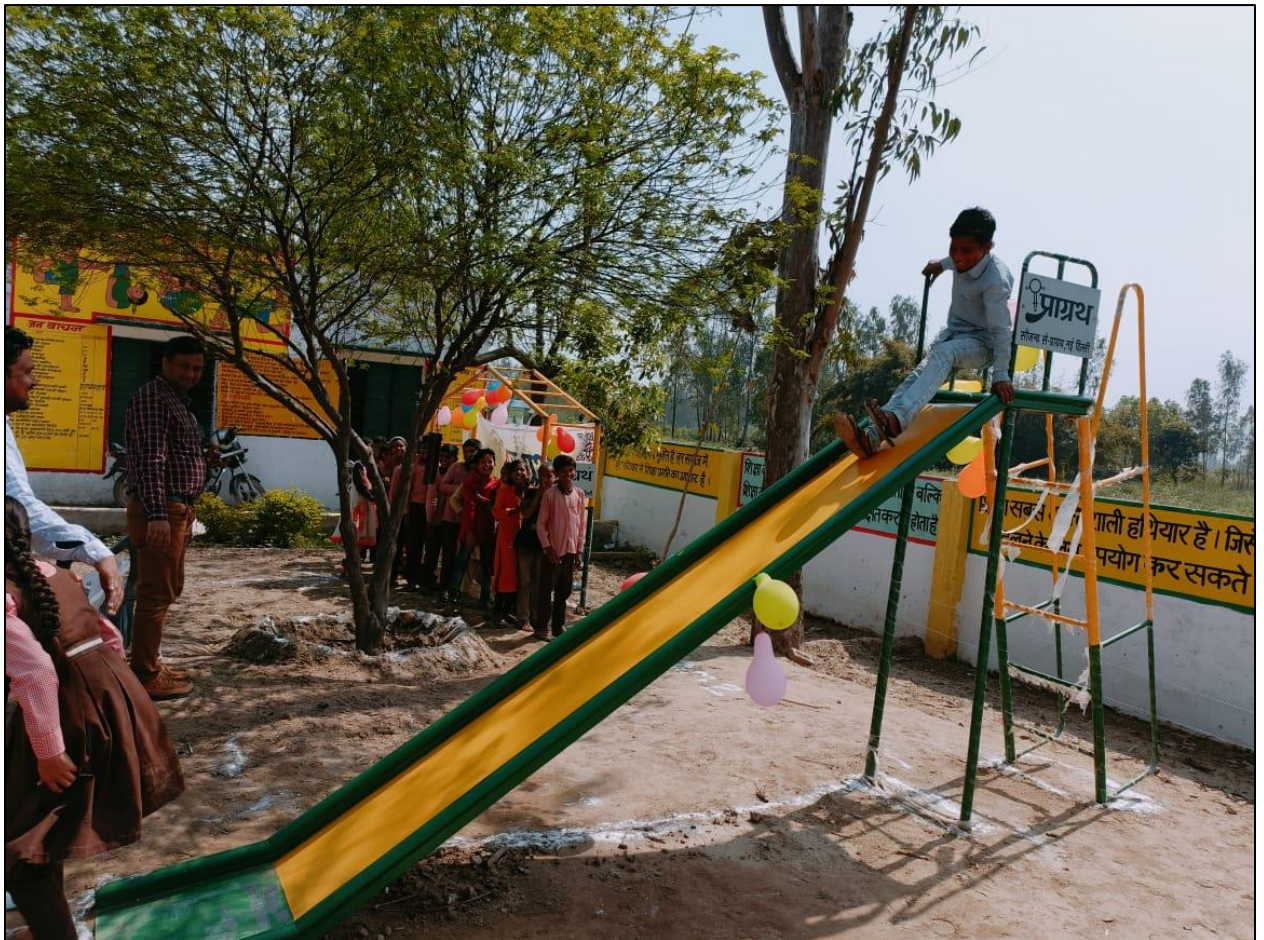
Pic 2: Installation of Slide at Primary School, Bamnauli, Bijnor, Uttar Pradesh
